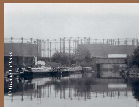
King's Cross Yard — Goods Way bridge
