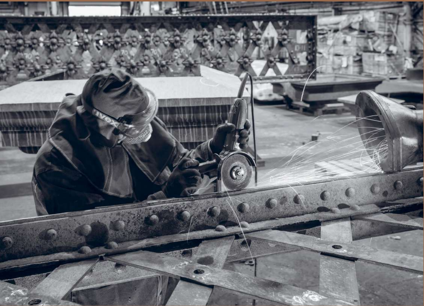
It has taken over two years to painstakingly refurbish the 123 cast-iron gasholders columns
