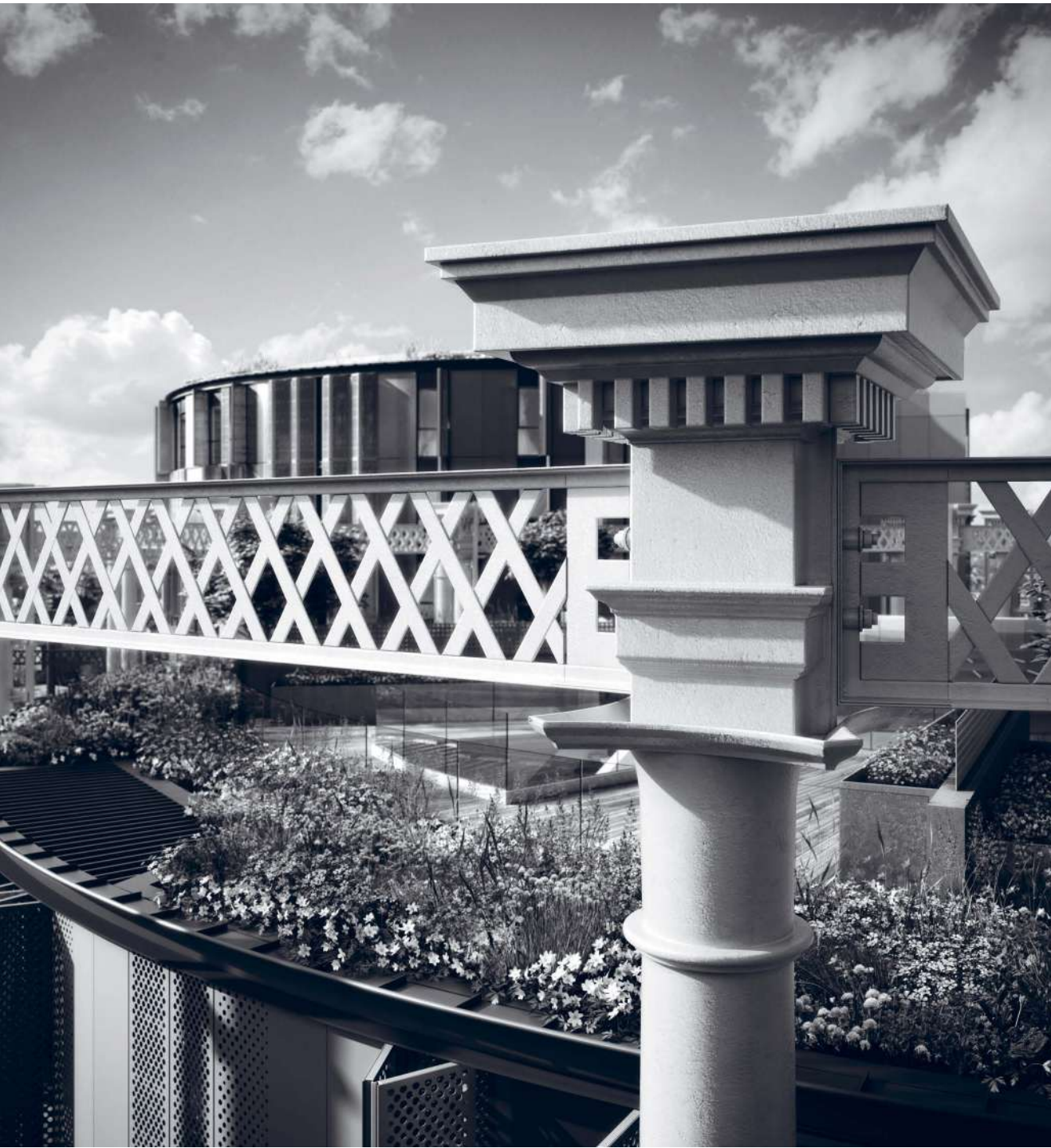
Gasholder 12 has a residents' roof garden designed by landscape design practice Dan Pearson Studio
