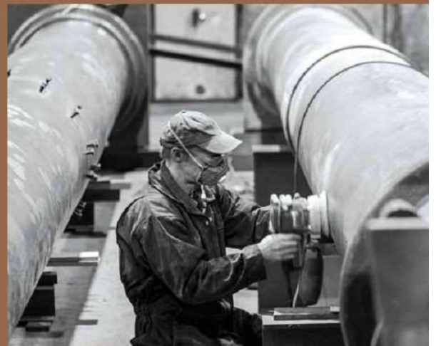
Highly skilled craftsmen in Yorkshire carefully refurbish the immense gasholder frames piece by piece
