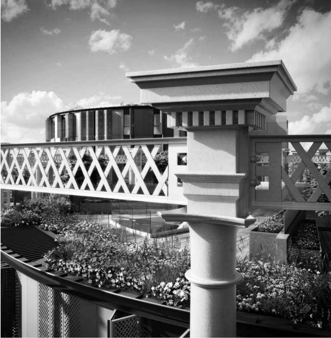
Gasholder 12 has a residents' roof garden designed by landscape design practice Dan Pearson Studio
