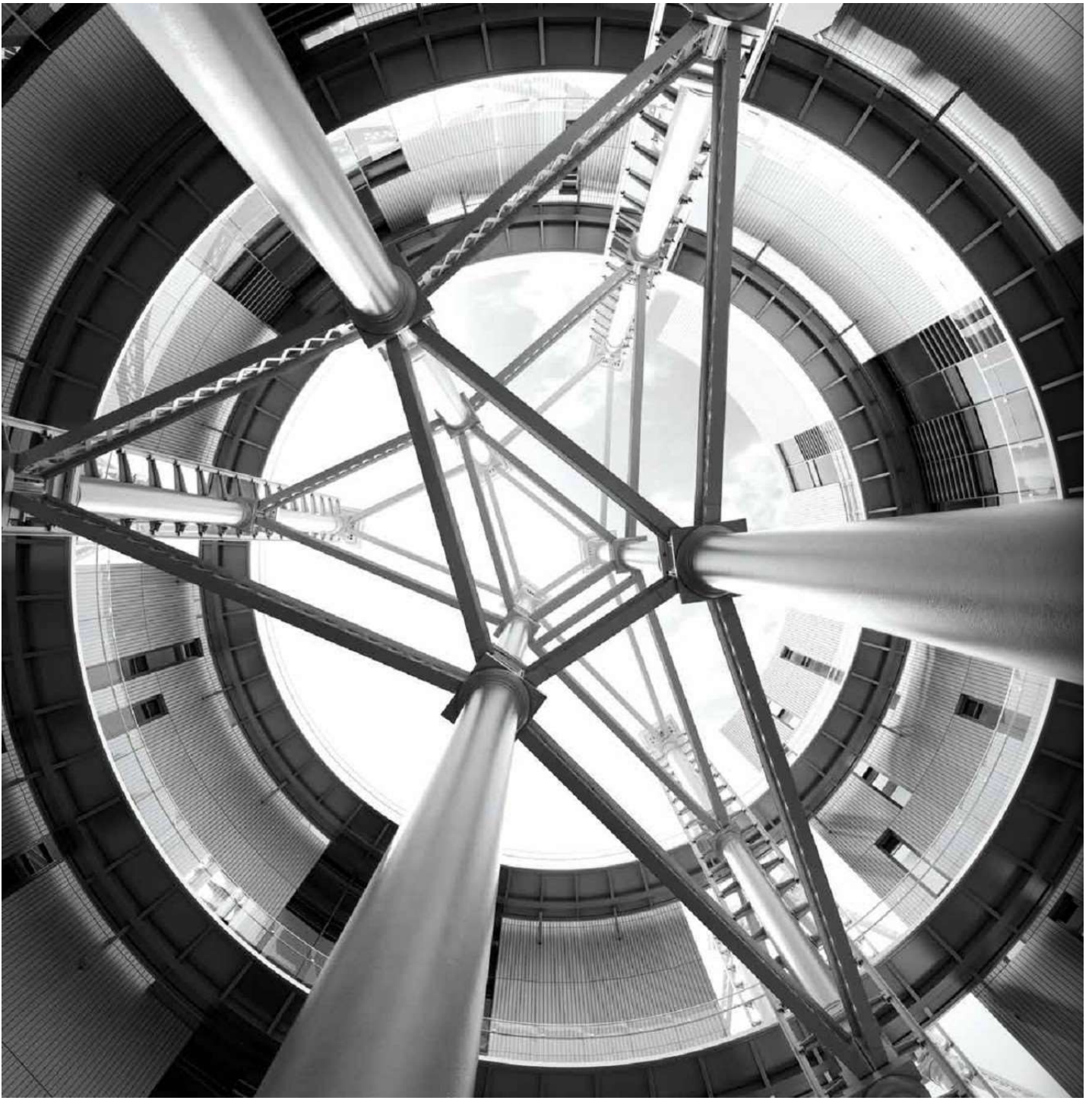
Looking skywards through the structure from within the central courtyard.
